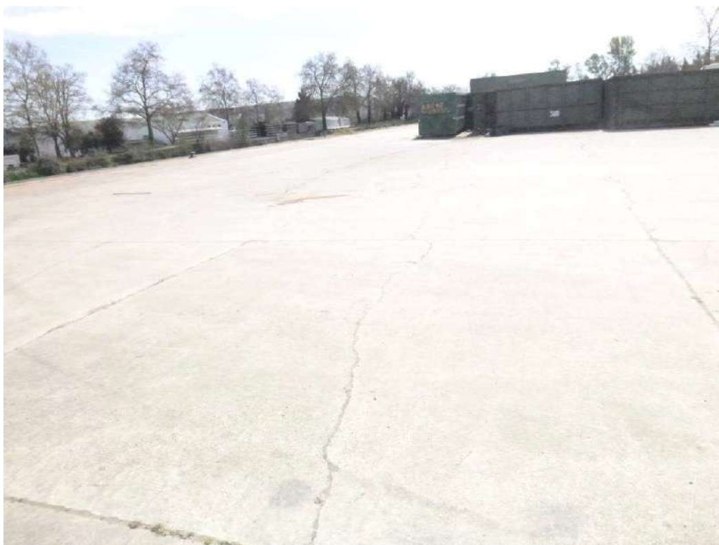
Figure 17 : Fissuration du dallage.
