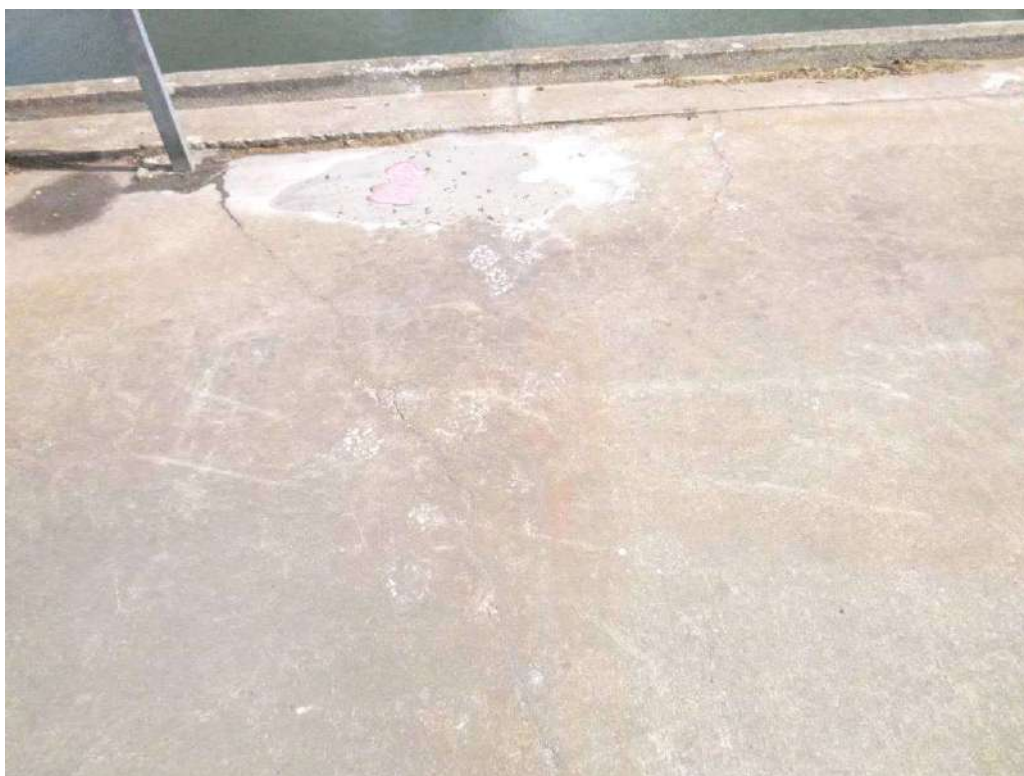
Figure 21 : Fissuration du dallage.
