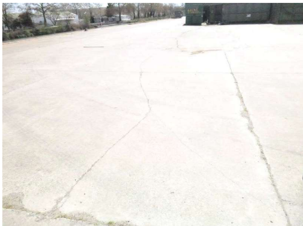
Figure 18 : Fissuration du dallage.
