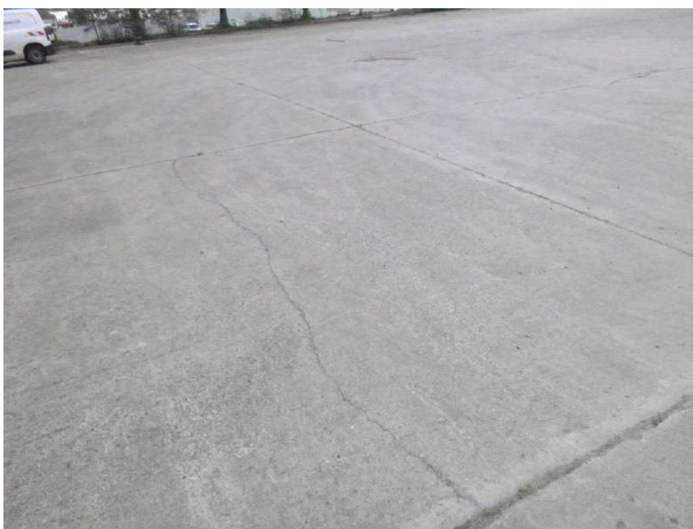
Figure 16 : Fissuration du dallage.
