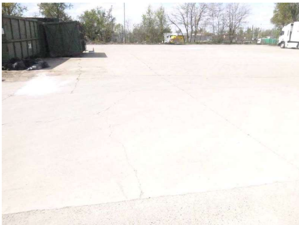
Figure 23 : Fissuration du dallage.
