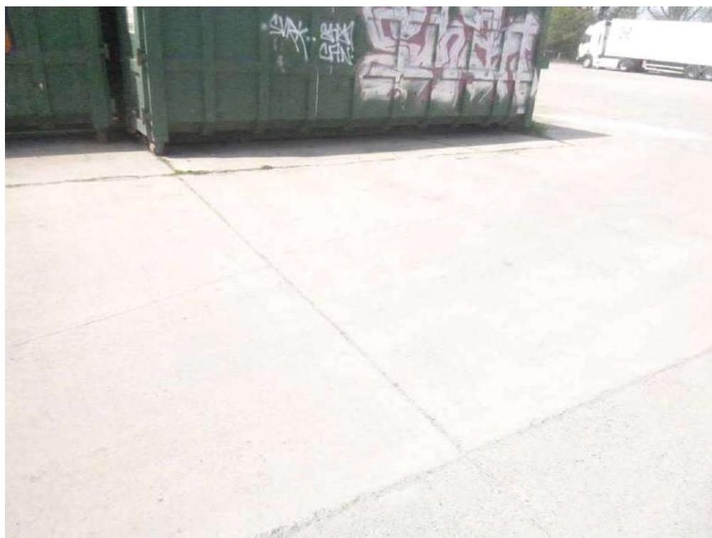
Figure 24 : Fissuration du dallage.
