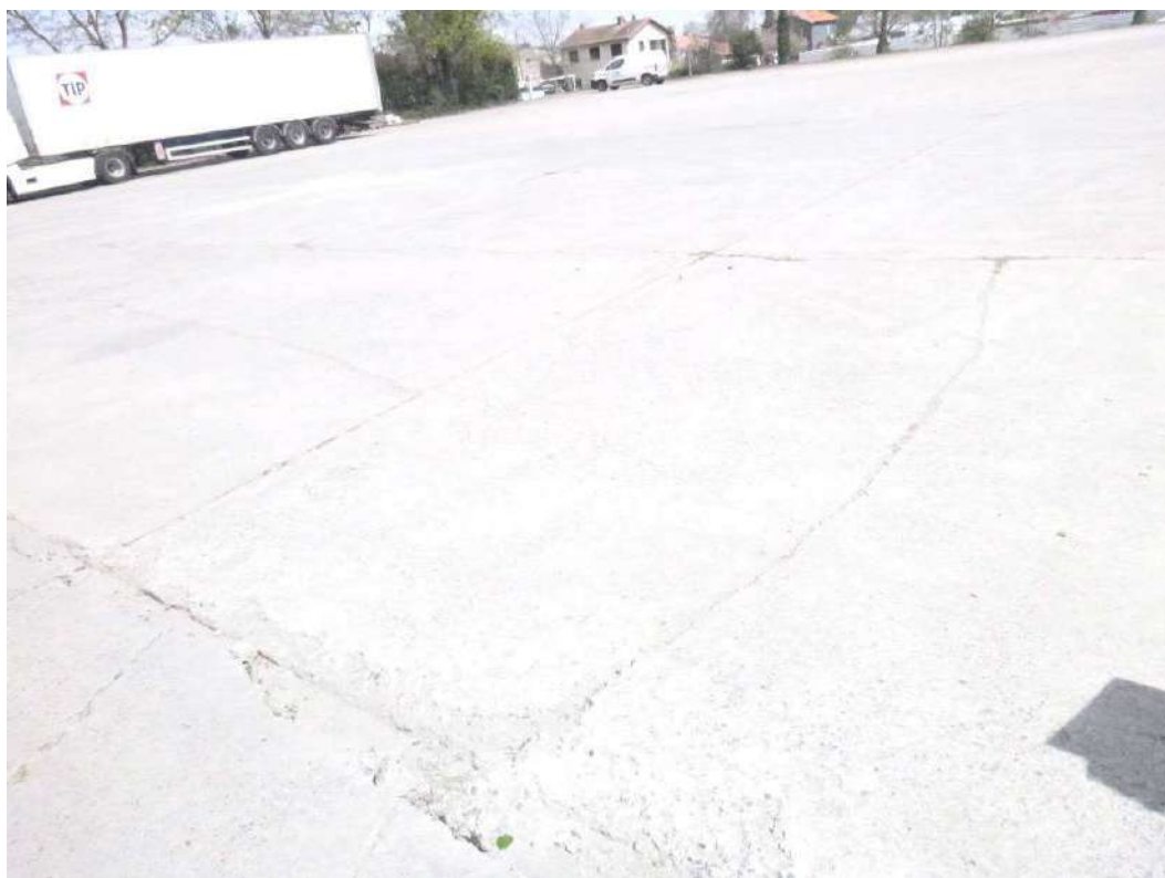
Figure 11 : Fissuration du dallage.
