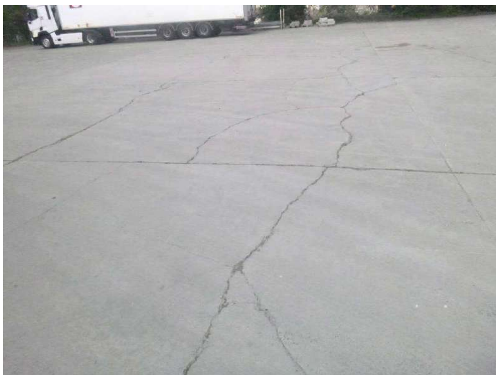
Figure 30 : Fissuration du dallage.
