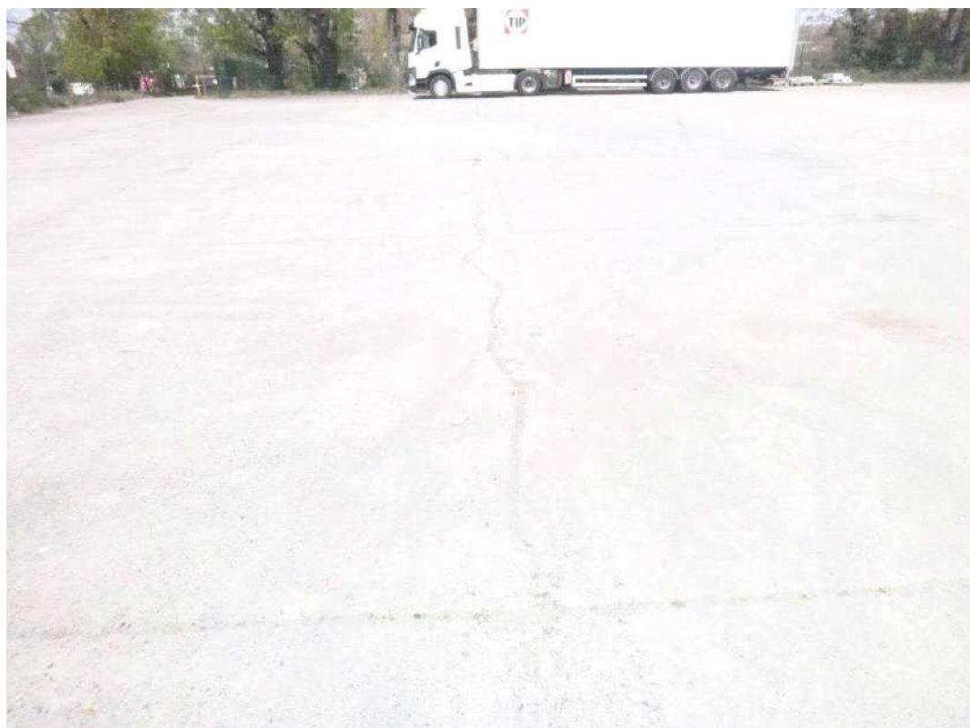
Figure 12 : Fissuration du dallage.
