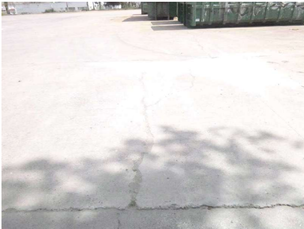
Figure 3 : Fissuration du dallage
