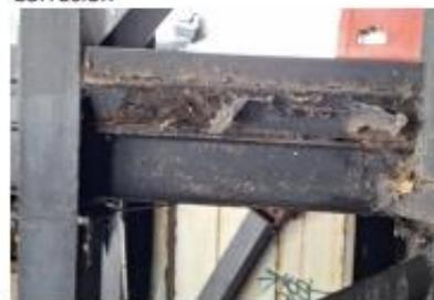
Corrosion charpente/bac acier/ assemblage
