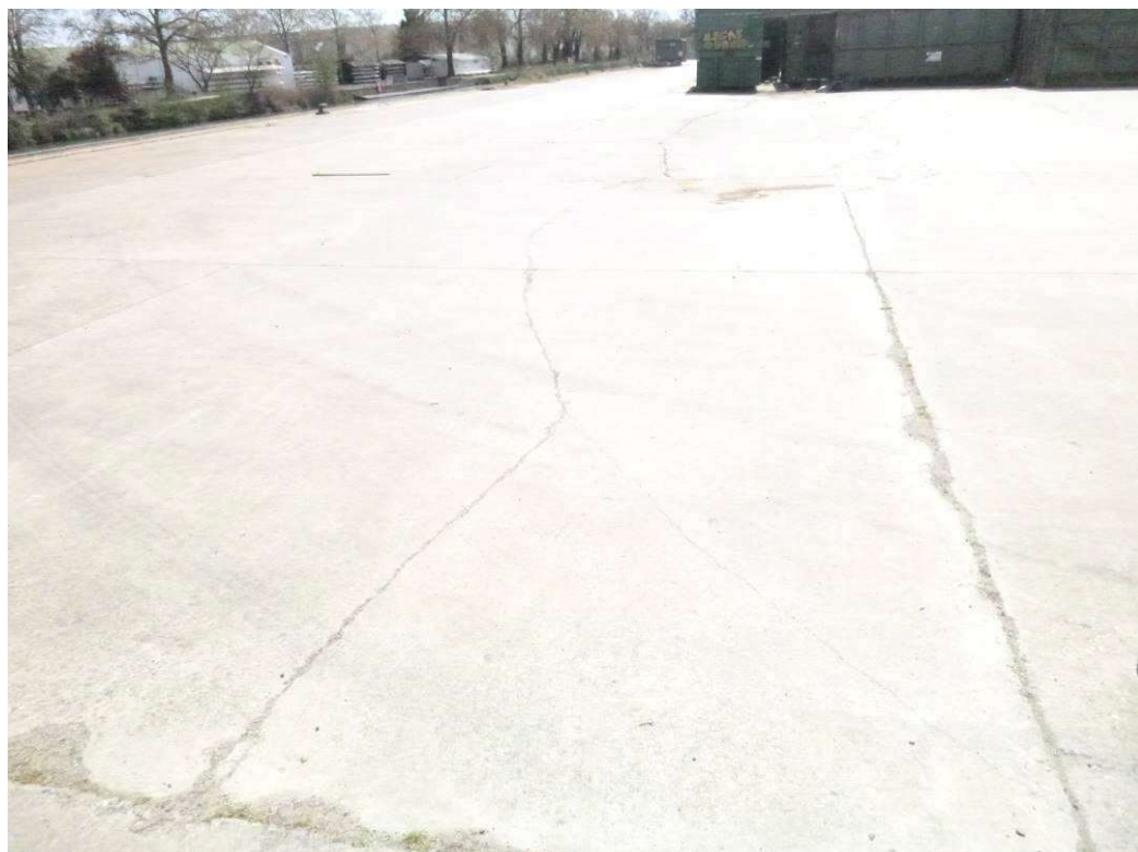
Figure 18 : Fissuration du dallage.
