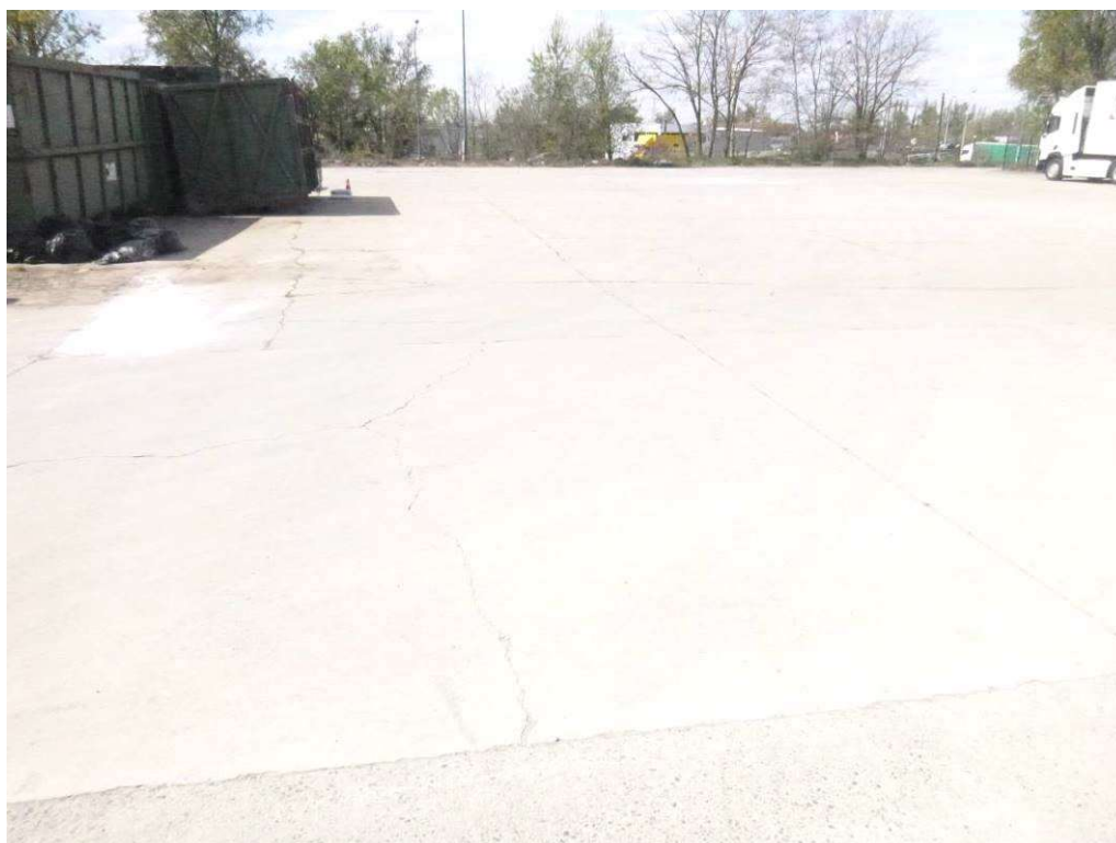
Figure 23 : Fissuration du dallage.
