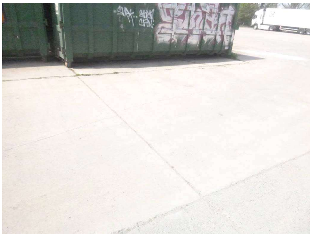
Figure 24 : Fissuration du dallage.
