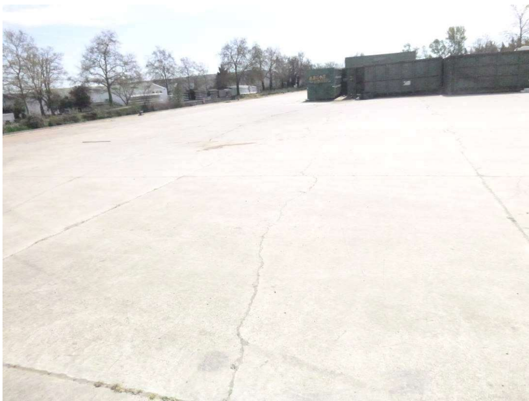
Figure 17 : Fissuration du dallage.
