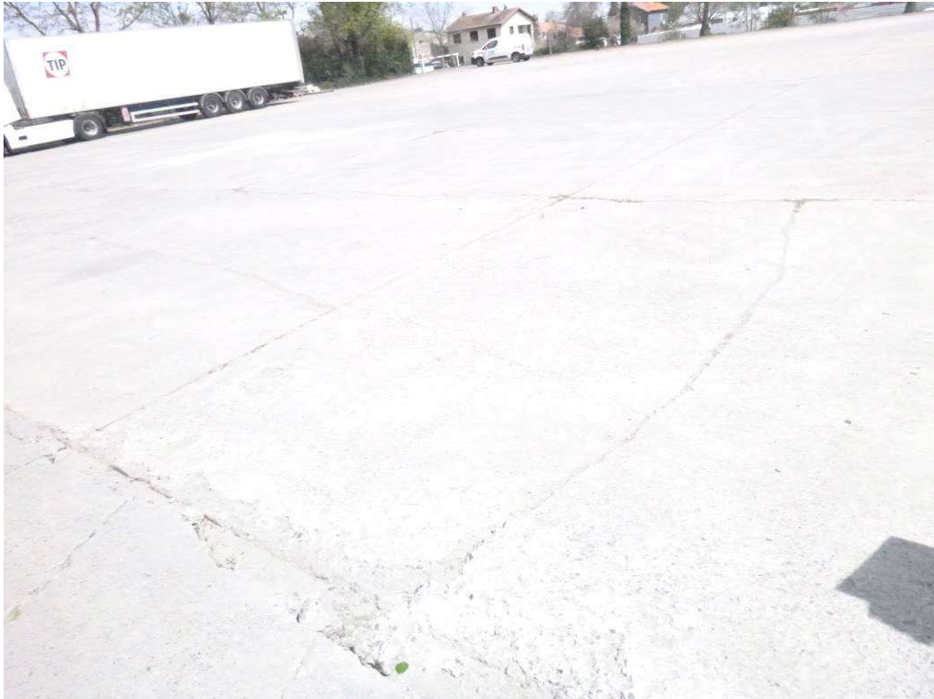
Figure 11 : Fissuration du dallage.
