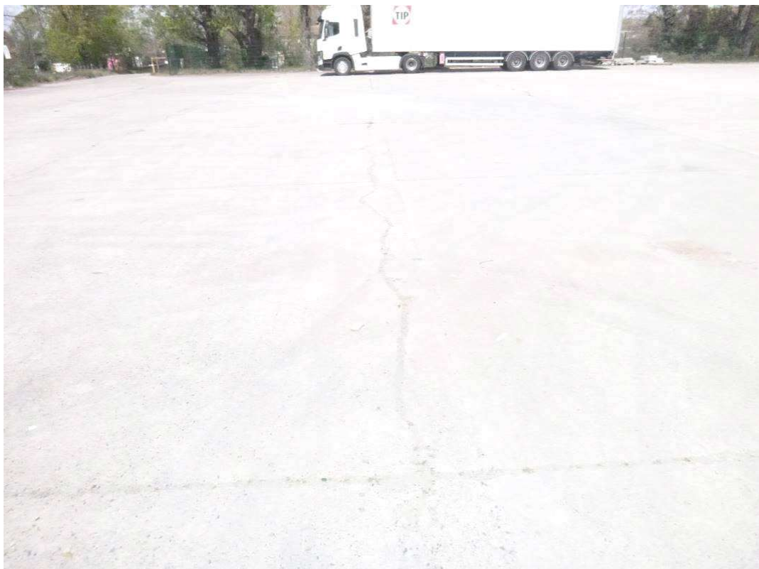
Figure 12 : Fissuration du dallage.
